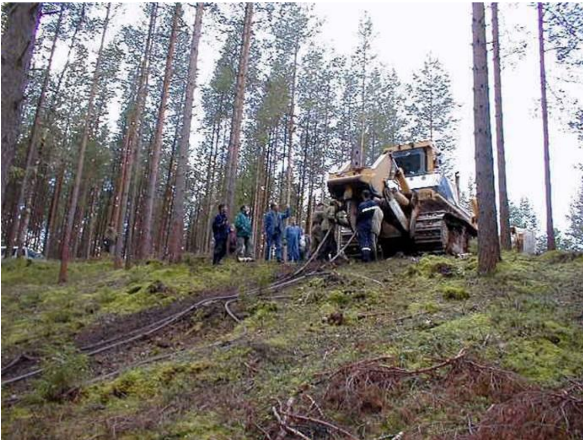
Preparing to pull it out.
